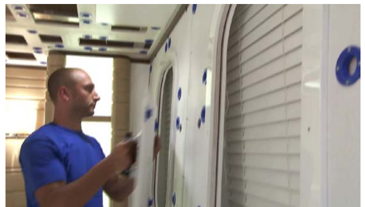
Filler Ring for Sure Catch Clips 2 mm thick. Part #43.CFIL 2 3/8" Outside Diameter
